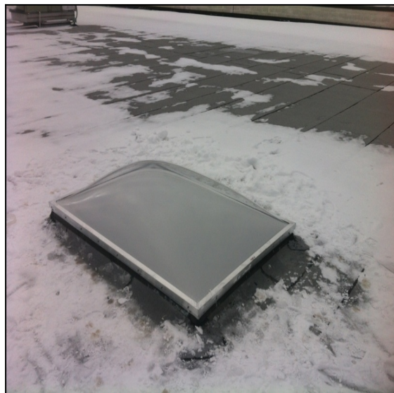
Photo 2 Notes: Installed new gasket at top of curb before installing new lens and fastening.
