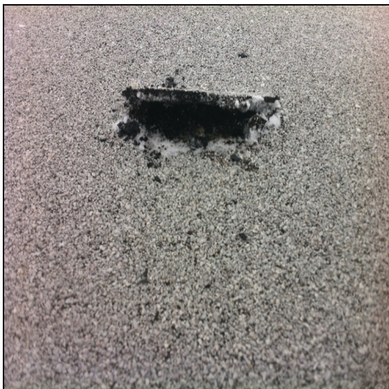
Photo 1 Notes: Found large puncture in roof's membrane. Removed snow, ice, and cleaned area.
