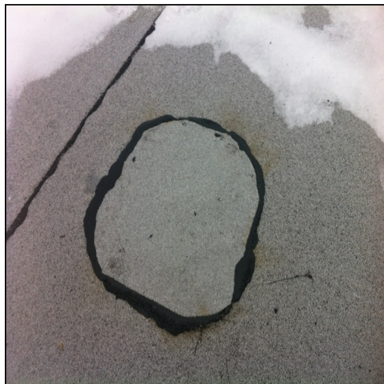
Photo 2 Notes: Installed white granulated modified to match existing roof system. All work completed per the manufactures specifications.
