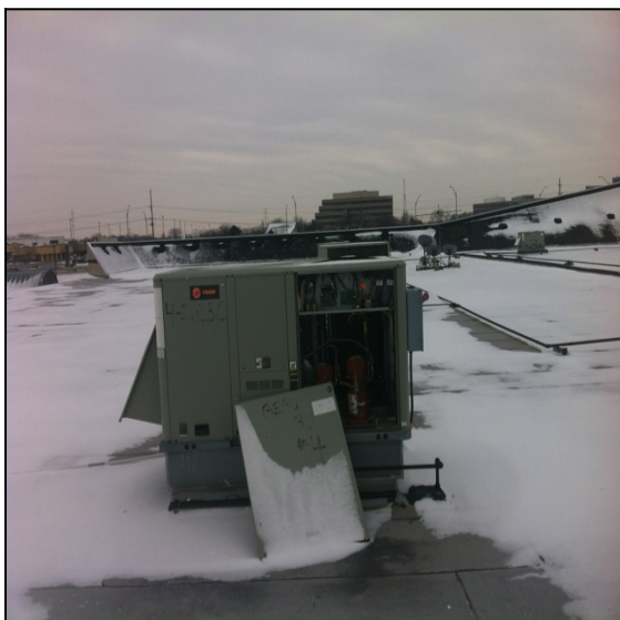
Photo 1 Notes: Due to severe winds Hvac unit door had blown off.
