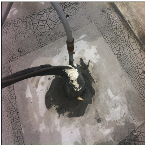
Photo 1 Notes: The asphalt has dried up and cracked open.
